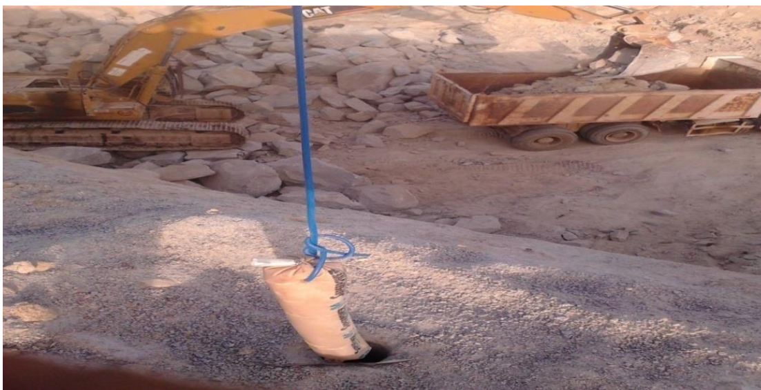
Figure 7: Priming of Holes for Primary Blasting
