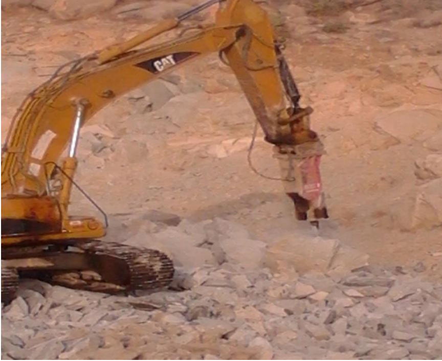
Figure 9: Rock Breaker attached to Power Excavator
