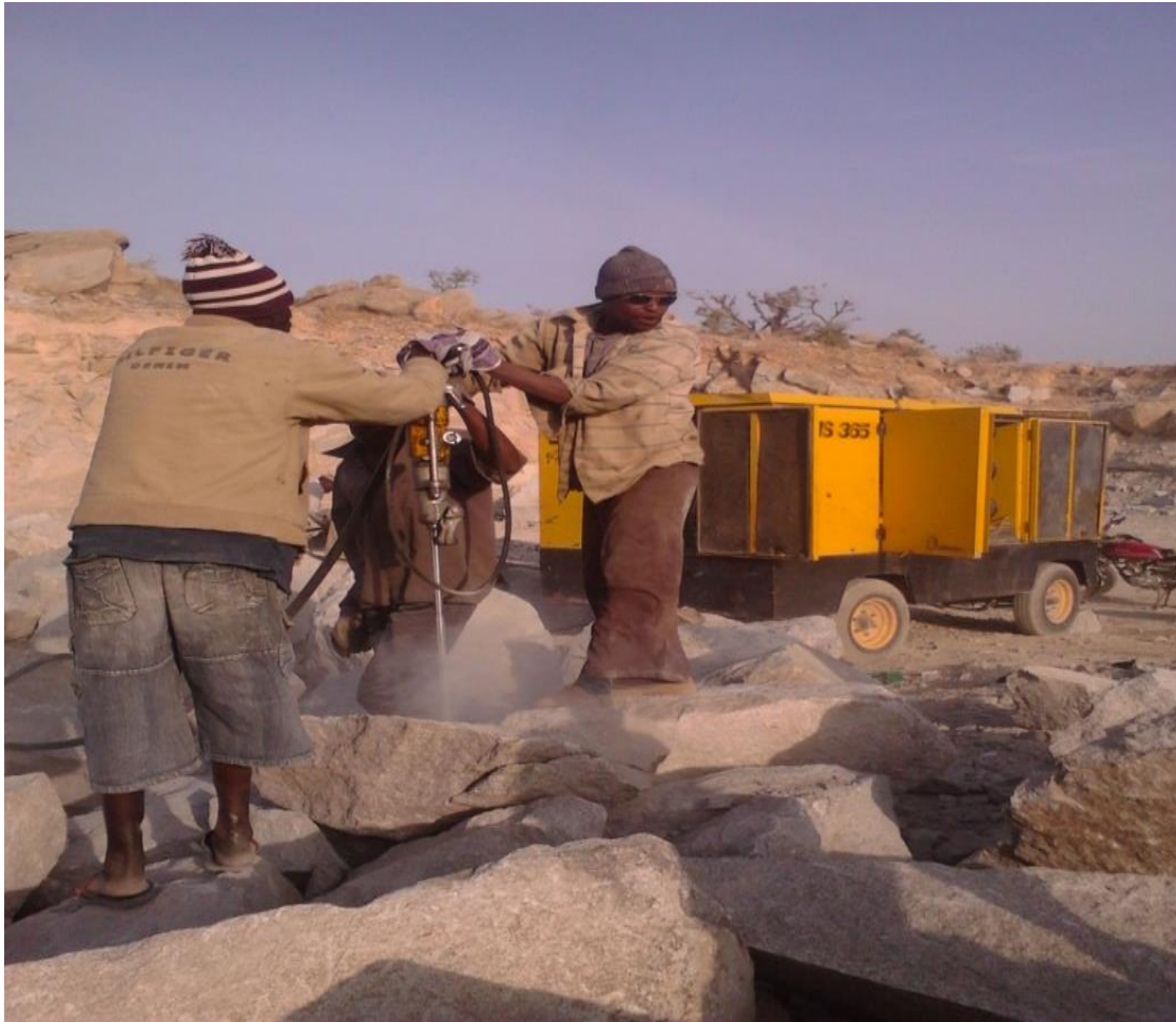
Figure 8: Handheld Drill (Jackhammer) Machine for Secondary Blasting
