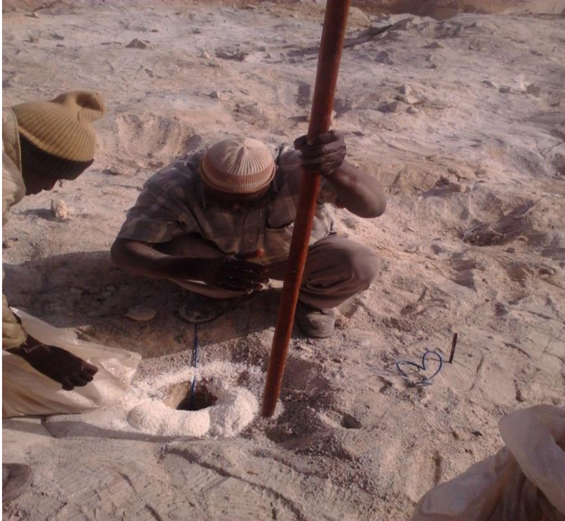
Figure 6: Charging of Holes for Primary Blasting
